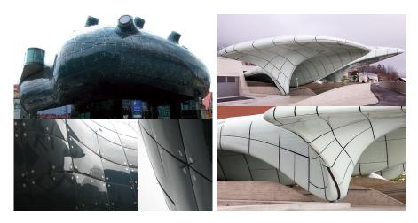
**Figure 2:** Projects involving double-curved panels where a separate mold has been built for each panel. These examples illustrate the importance of the curve network and the existing difficulties in producing architectural freeform structures. (Left: Peter Cook and Colin Fournier, Kunsthaus, Graz. Right: Zaha Hadid Architects, Hungerburgbahn, Innsbruck.) Figure taken from [Eigensatz et al. 2010].
